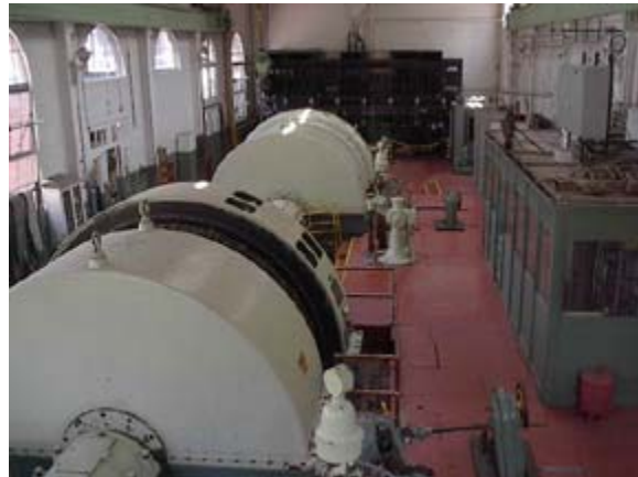
Flowing water spins a turbine, which in turn spins an electrical generator to produce electricity.
