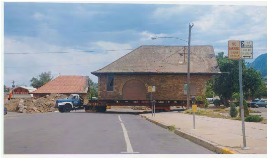
Figure 2 Depot being moved from original location in 1973
