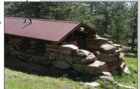
Completed repairs to the 1935 CCC Halfway House
