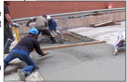
Concrete work at the 14th & Walnut Parking Garage
